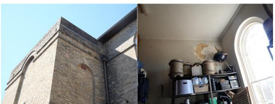
Suggest copings are removed and re-bedded in mortar to prevent furter water ingress. Could be re-designed to create a water drip to reduce the likelihood of water running down the face of the wall and top section of brickwork repointed in air/hot lime mortar. A specification / detail can be supplied if requested.
