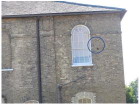
Appears to be a previous core drilled hole in the masonry which need a brick carefully cutting and inserting with air/hot lime mortar.
