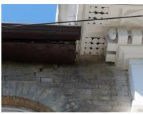
There appears to be (historic) dark water to the brickwork from the end of the gutter abutment to the mouldings, this will need to be checked to see if it is indded, historic, or a current issue.
