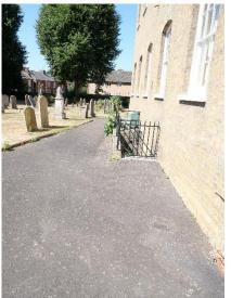
Note - suggest altering the tarmac so there is a drainage gap/gravel abutment to the masonry to reduce rainwater splashback. A specification / detail can be supplied if requested.
